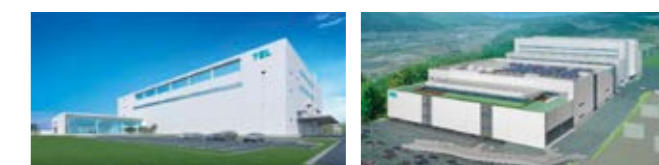
Tokyo Electron Technology Solutions New Production Buildings (Left: Tohoku Plant Right: Fujii Plant)
