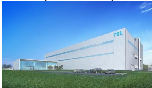
Oshu City, Iwate Prefecture: approx. ¥13.0B construction cost (Began construction in October 2018, completion scheduled for September 2019)
