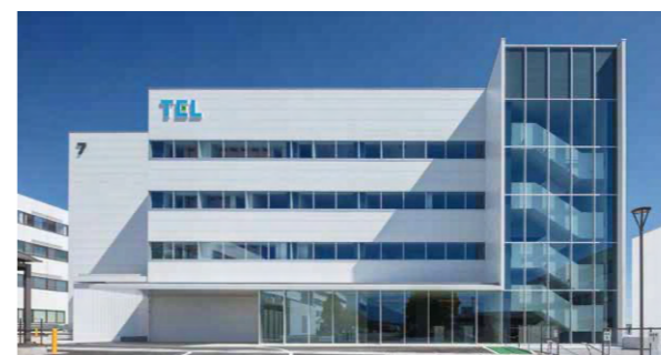
New Development Building Completed in July 2023 (Nirasaki City, Yamanashi)
