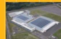
Tokyo Electron Miyagi new plant
