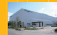
Tokyo Electron Kyushu new production building
