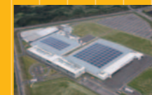
Tokyo Electron Miyagi new plant
